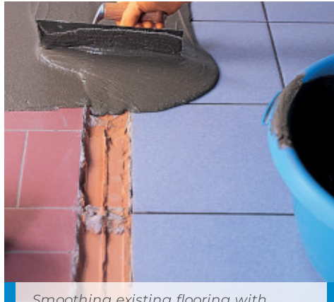
Smoothing existing flooring with Adesilex P4
