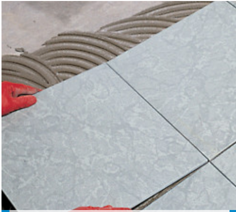
Laying porcelain tiles
