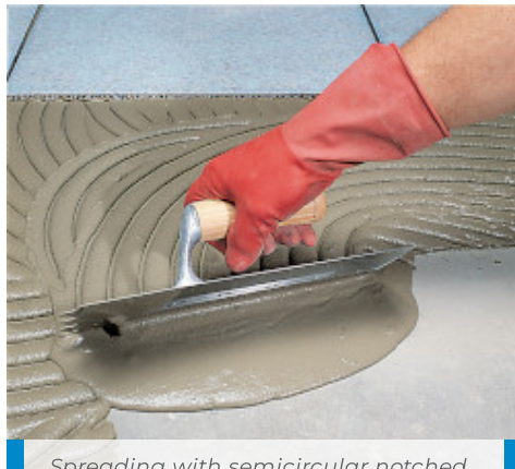
Spreading with semicircular notched trowel
