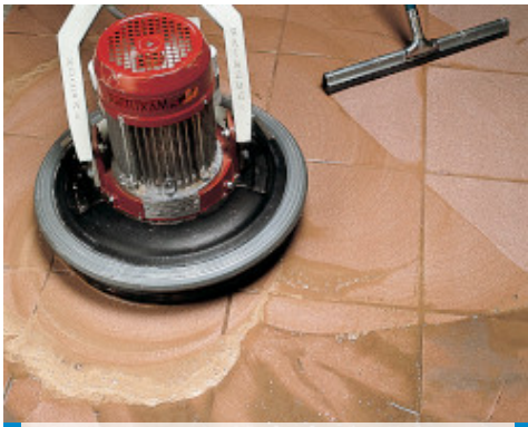
Finishing a porcelain tiled floor with single-brushed power float or rubber squeegee
