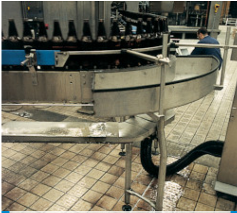
An example of a grouted brewery floor
