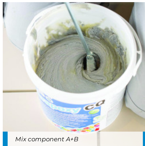
Pour the hardener (component B) in the container of component A
