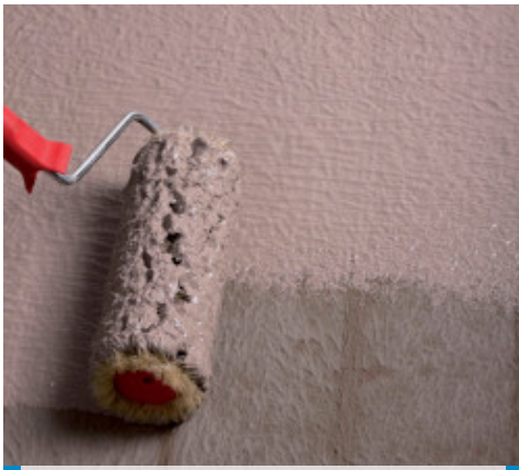
Waterproofing of details by roller
