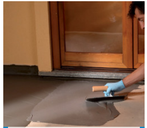
Waterproofing of terraces by trowel
