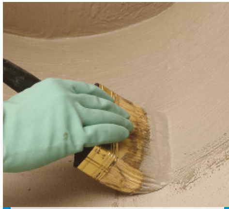
Waterproofing of details by brush
