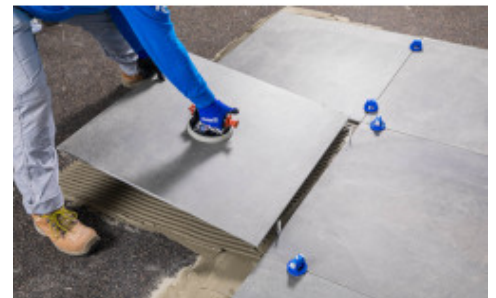
Spread the adhesive on the Mapesonic CR and bond the new floor finish
