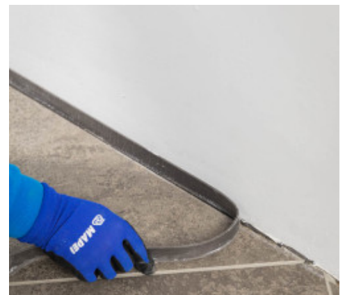
Spread the adhesive on the Mapesonic CR and bond the new floor finish
