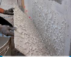
Checking the back face of the tile if it is completely buttered when laying on an external façade
